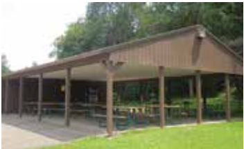
Sycamore Creek Park Pickering Shelter 300 Covered Bridge Lane (Seats approx. 80)
